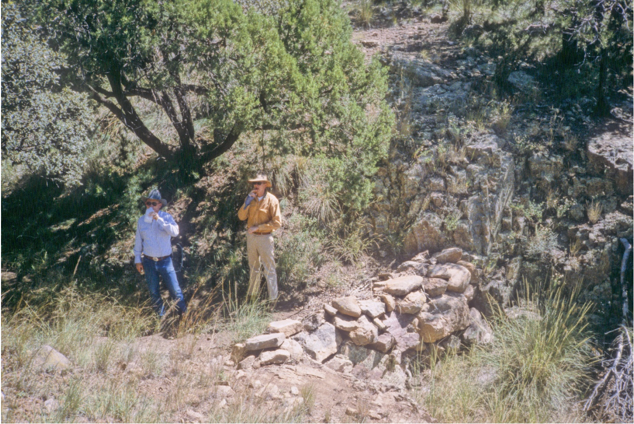
Figure 1. Loose rock dam on Joe Austin ranch 1993. Note size of rocks, size of dam and bedrock on both sides of channel. Larry Humphrey and Joe Austin in photo.
